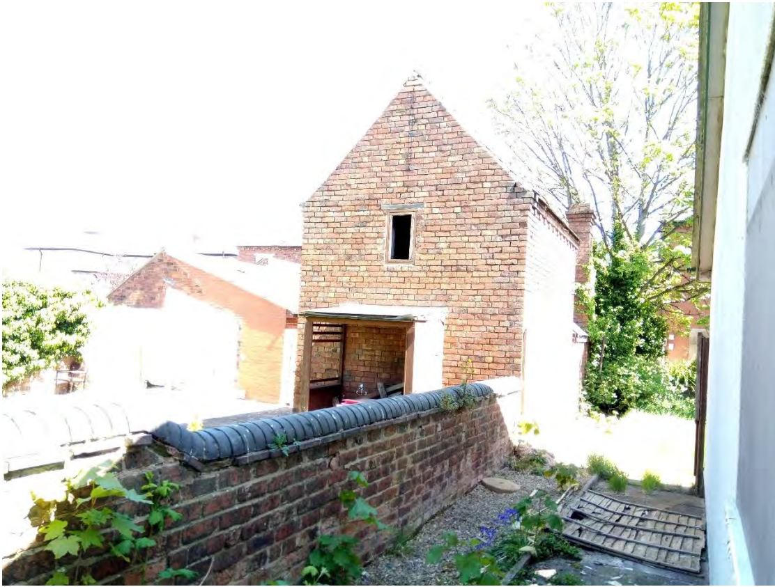
22.7 Rear of application property, including neighbouring property of 41 Wood Green Road on the left.
